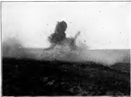
Blowing up of the Oliphant River bridge.
